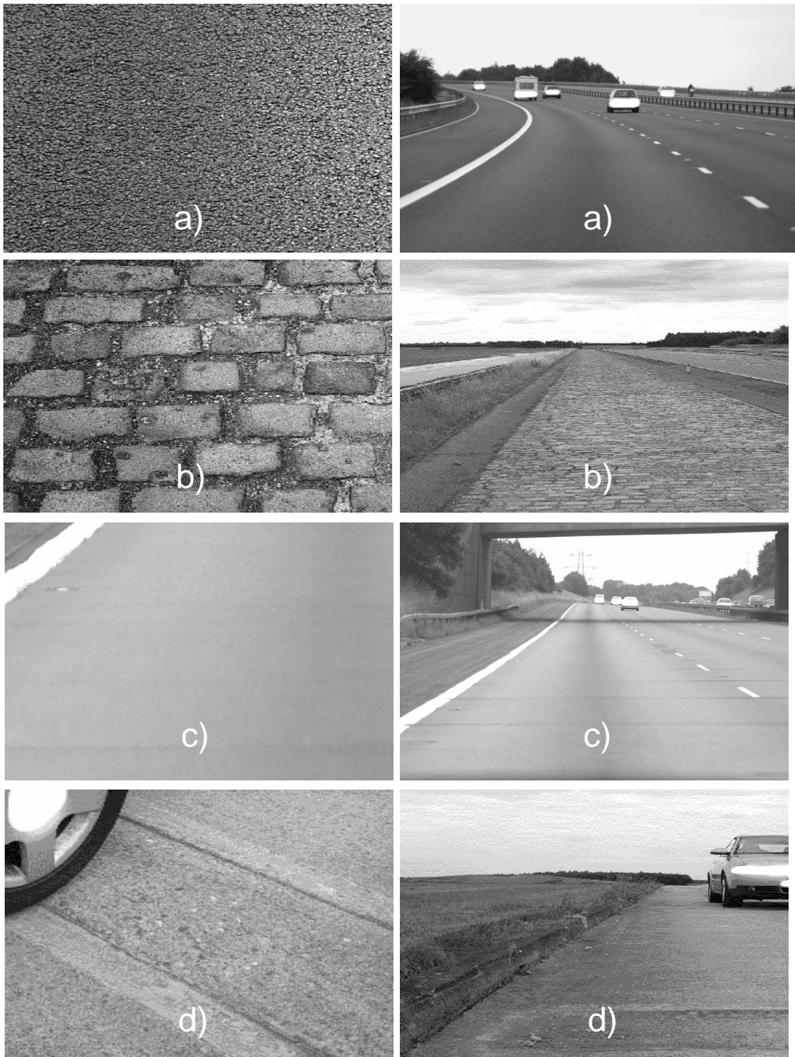
Figure 3 Road surfaces which produced the steering wheel acceleration time histories used in the laboratory experiments.
