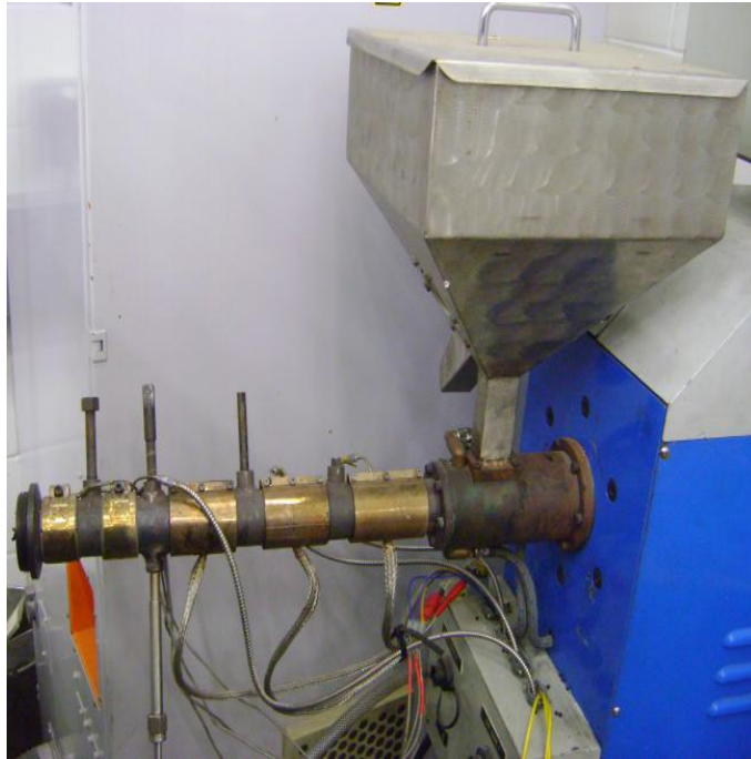
Figure 3-8: heating bands of the barrel (left) and power distribution box for heaters and thermocouples.
