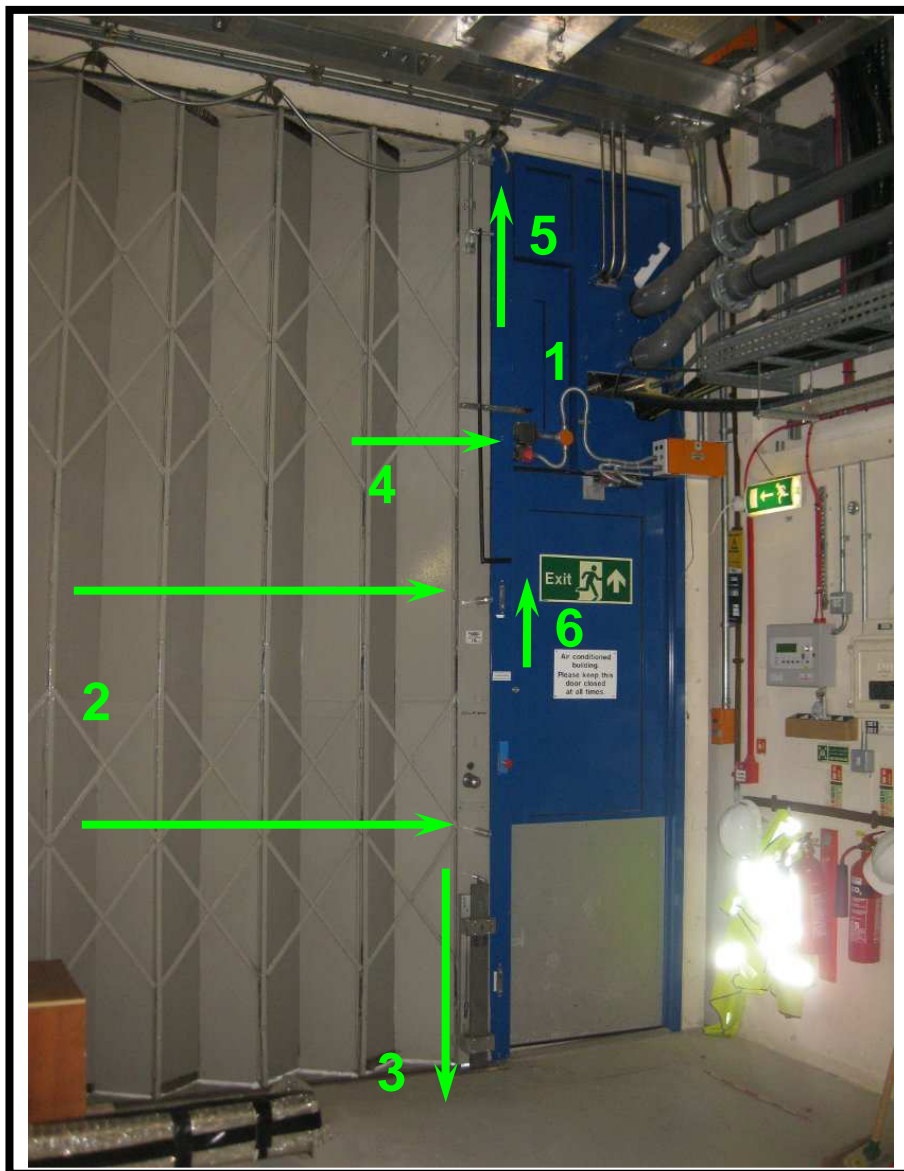
Figure 4.2.5: Closing the Equipment Door.
