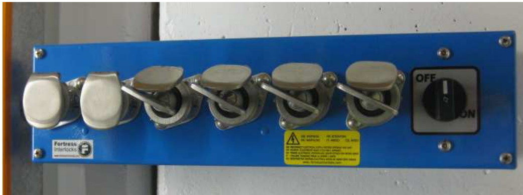
Figure A2.1: DSA Roof Keyswitch
