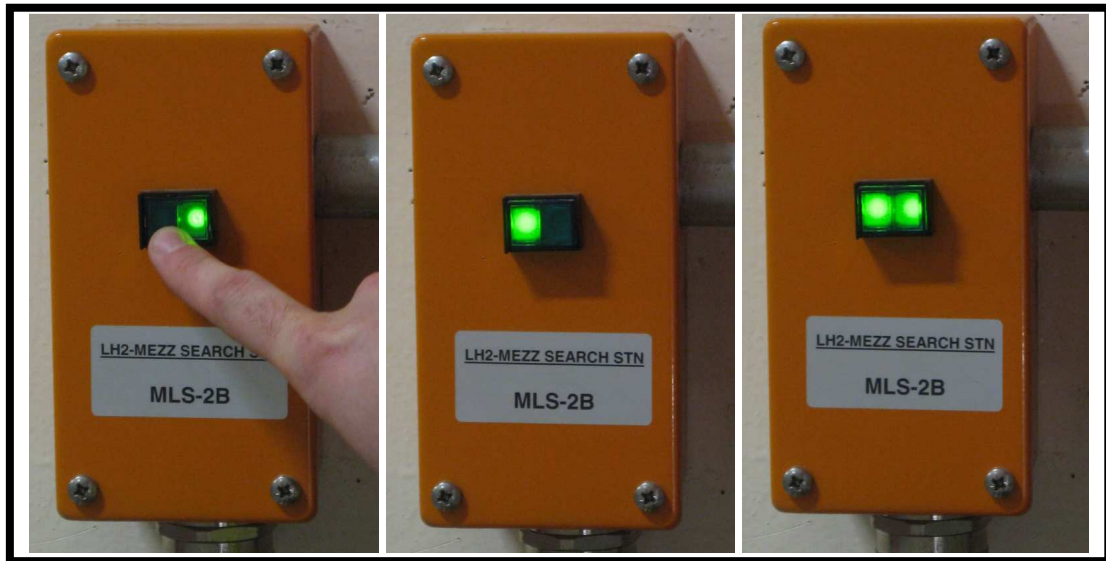
Figure 4.3.1: Search Point Sequence: this button (2B) pressed (left); remote button (2A) pressed (centre); search point made (right).
