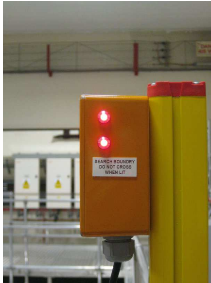
Figure 4.3.3: Light Curtain Active warning indicators
