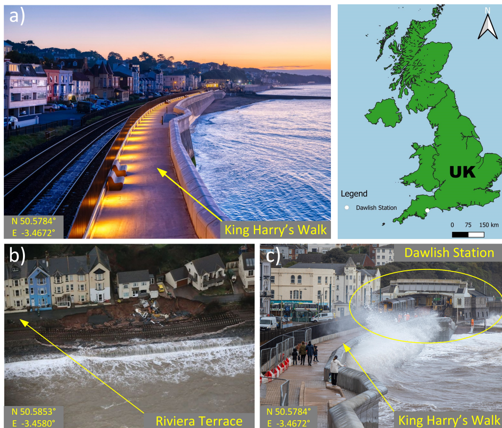
Figure 5.1: Location of Dawlish railway station. a) The completed section of the new seawall looking towards the train station along King Harry's Walk. b) An aerial view of the seawall damage sustained at Riviera Terrace in February 2014. c) Waves impacting the newly constructed seawall south of the station, now 2.5m taller with an integrated wave return. ©Network Rail.[92]
