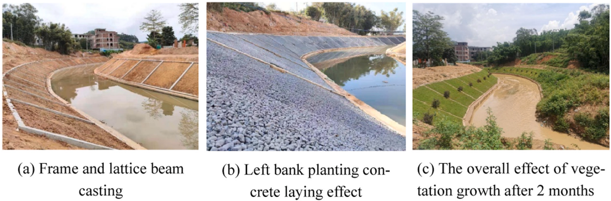
Fig. 28. Construction progress of river slope protection.
