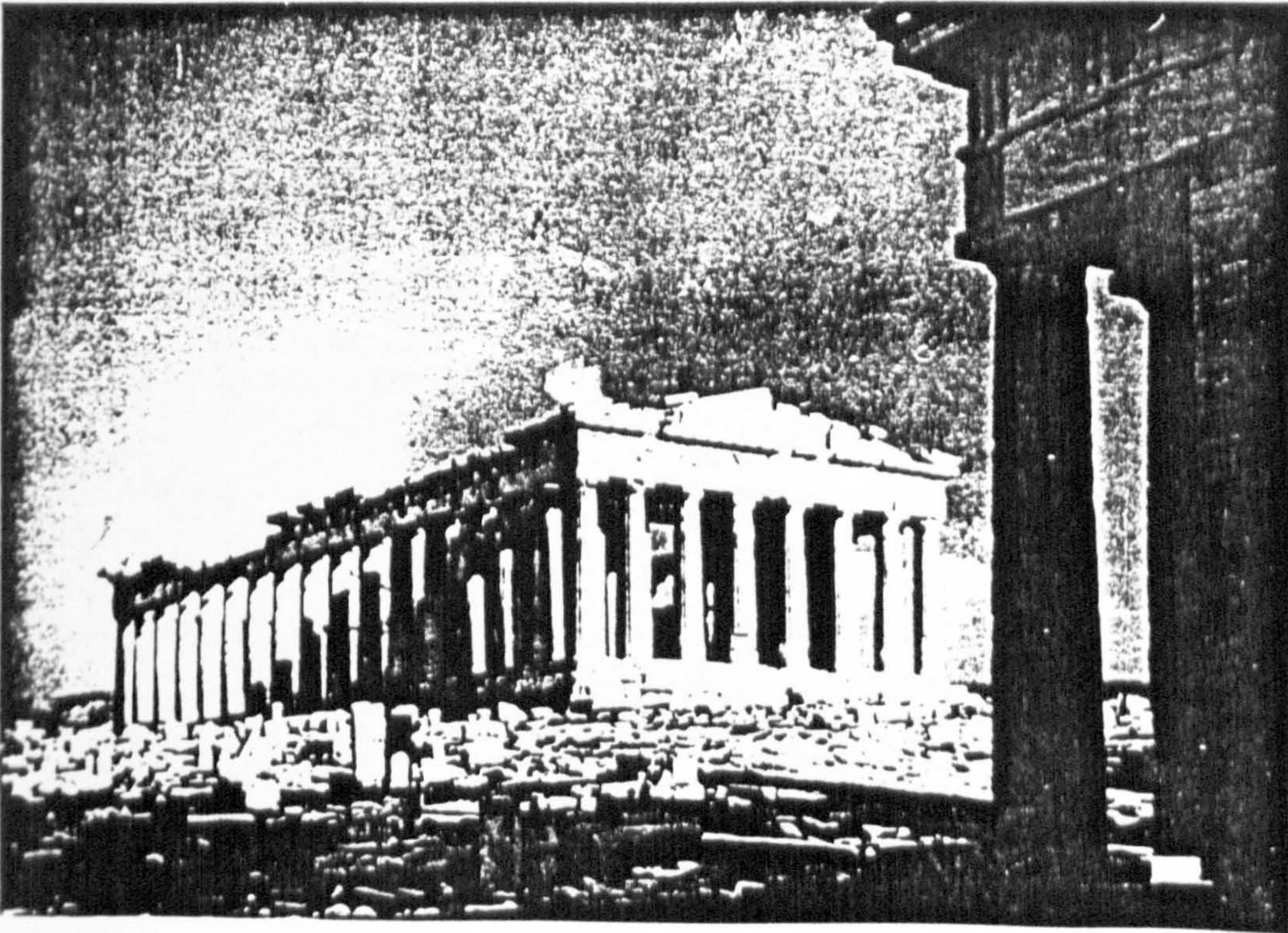
A.2.iv The Parthenon, Athens, View from Ground Level
