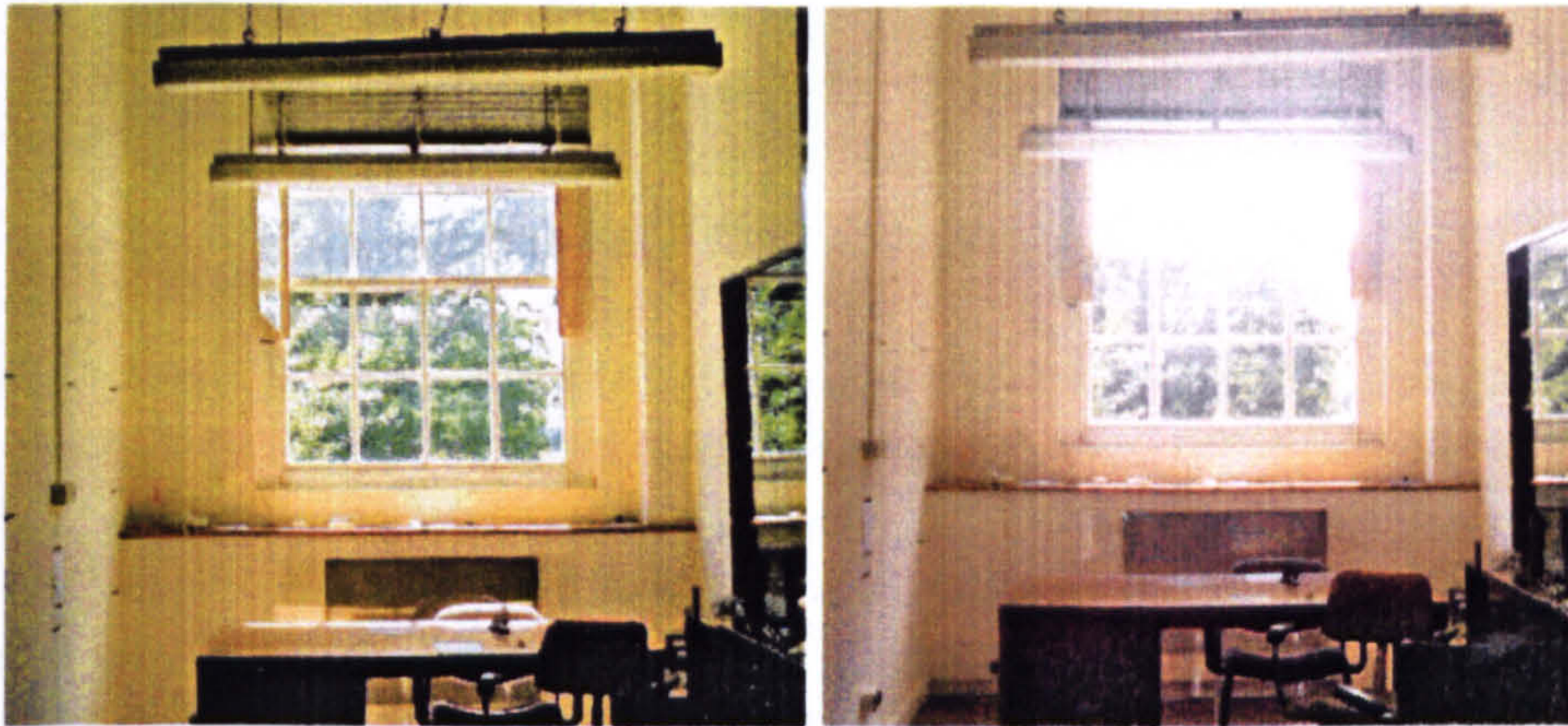
Fig 1: (Left): A traditional window. (Right) A window with the top third coated in microprisms.
