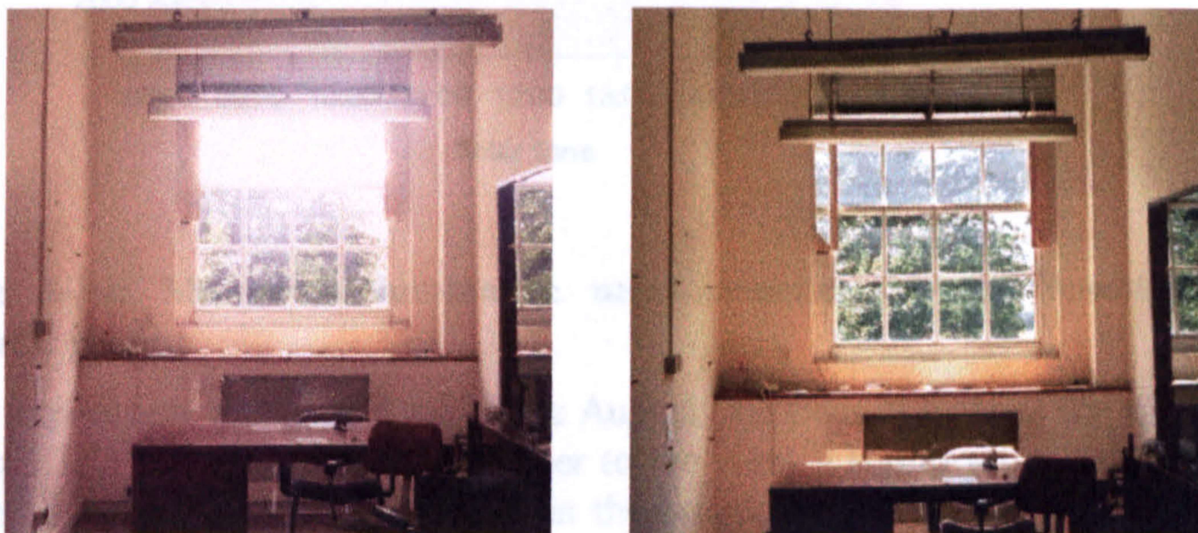
Fig 3-17: (Left) Prisms on office window at solar noon. (Right) Office window without prisms at solar noon. Exposure for both photographs: f/11, 1/60s, 100 ASA.
