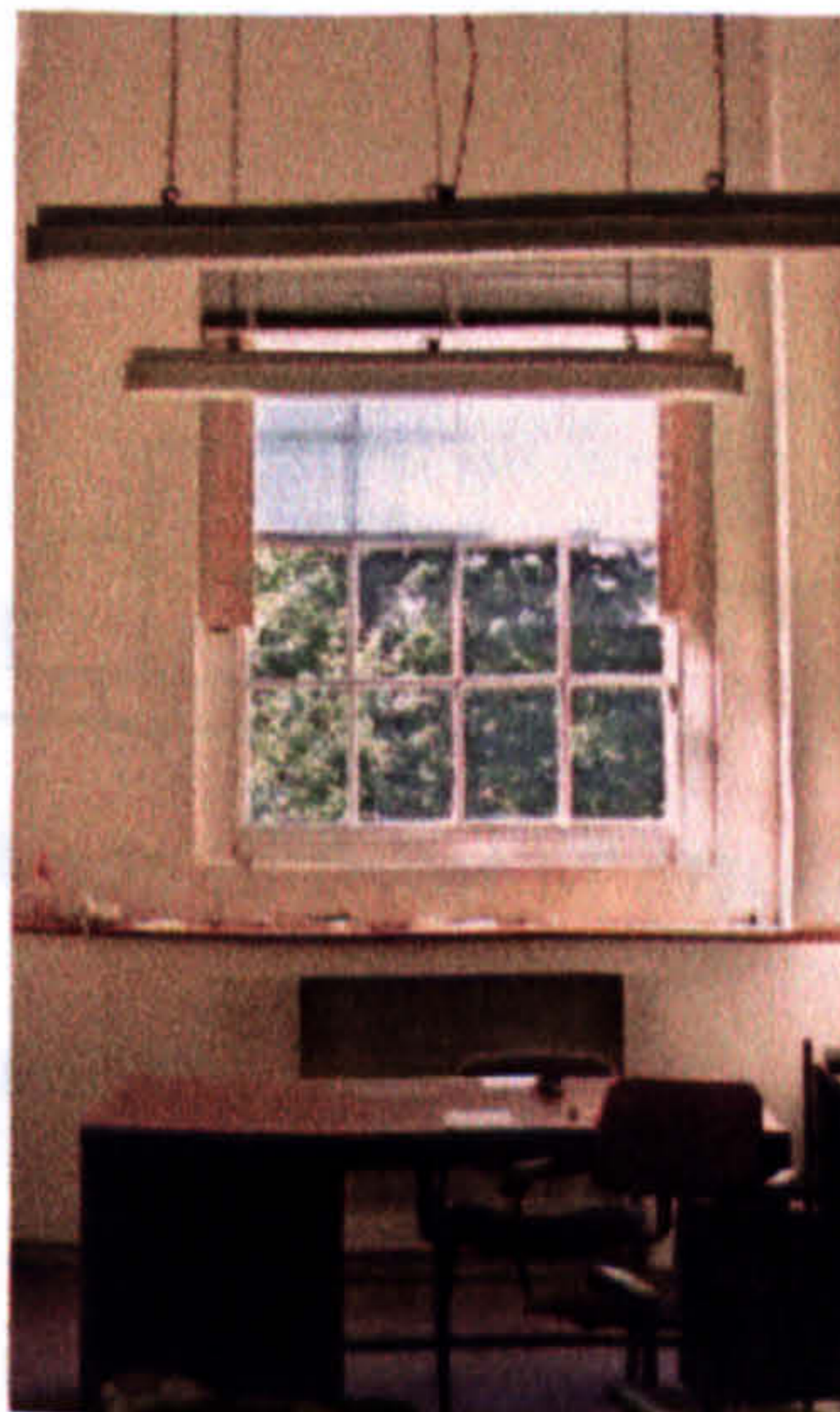
Fig 3-7: Prism array over an office window at NPL (exposure: f11, 1/60s, 100 ASA).
