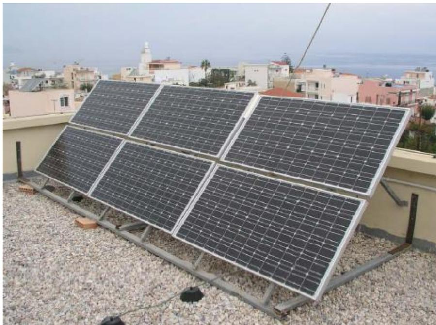
**Figure 4-1:** The six module PV array.
