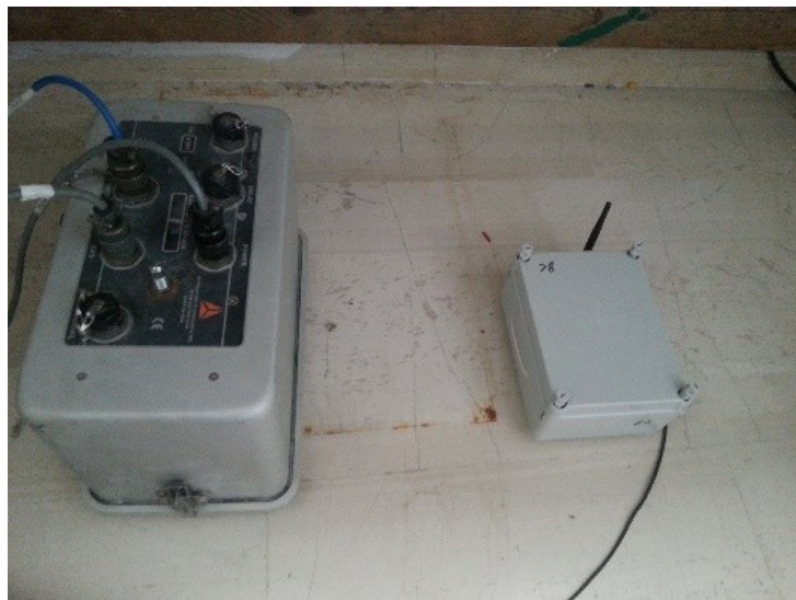
Figure 3.20. RefTek 130-SMA (left) and Wasp mote (right) installed (with screwing) on the second floor of the old building of TEI of Crete at Chania.
