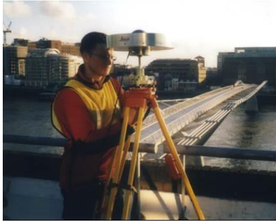
Figure 12, The Leica GR530 GPS receiver and Choke Ring antenna reference station being set-up adjacent to the Millennium Bridge [Roberts et al. , 2004].
