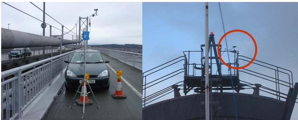
Figure 21, The Omni Instrument weather station placed at location F (left) and the Leica AT502 GPS antenna located at location A2 (right) on the Forth Road Bridge [Roberts et al. , 2012].
