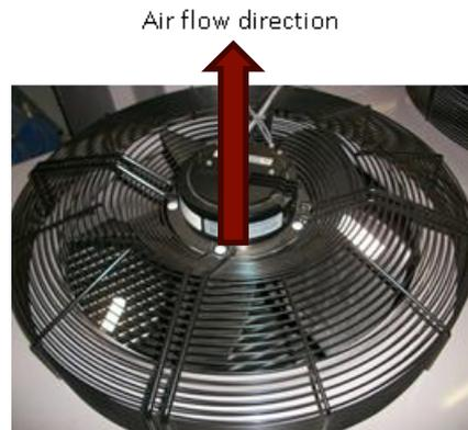
**Figure 3.17 Gas cooler main fan**
