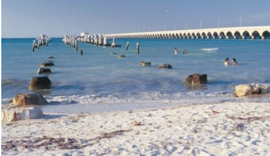
Figure 1 Progreso Pier, Mexico – the pier in the background was constructed in 1940 and used stainless steel reinforcing bar whereas the pier in the foreground was constructed in 1969 and used carbon steel reinforcing bar (Courtesy of the Nickel Institute)
