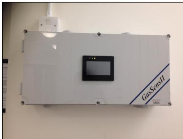
**Figure 3.2, Hydrogen Sensor Box installed in the entrance of the Hydrogen Lab**
