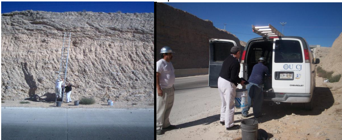
Photo 1 Camino real road left cut bridge 2 Cementera ; Photo 2 similar to photo 1
