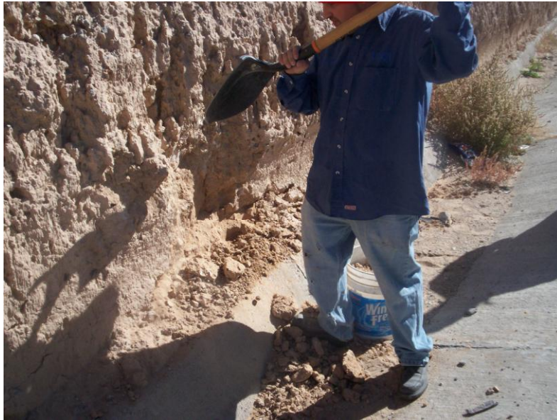
Photo 3 Lower Strata 1 point 5 windy sand C.R. 10+800
