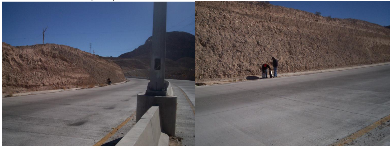
Photo 1 km 10+800 Camino real strata 1 windy sand conglomerate in the middle and windy sand lower strata
