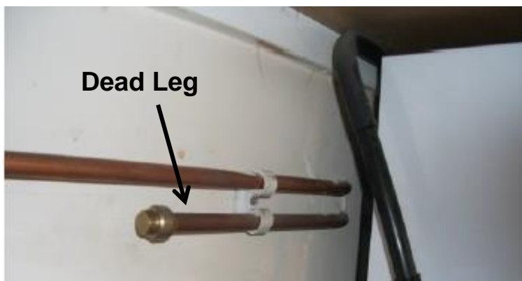
Figure 2.5: Photographs showing a dead-leg (Ibbotson, 2011).
