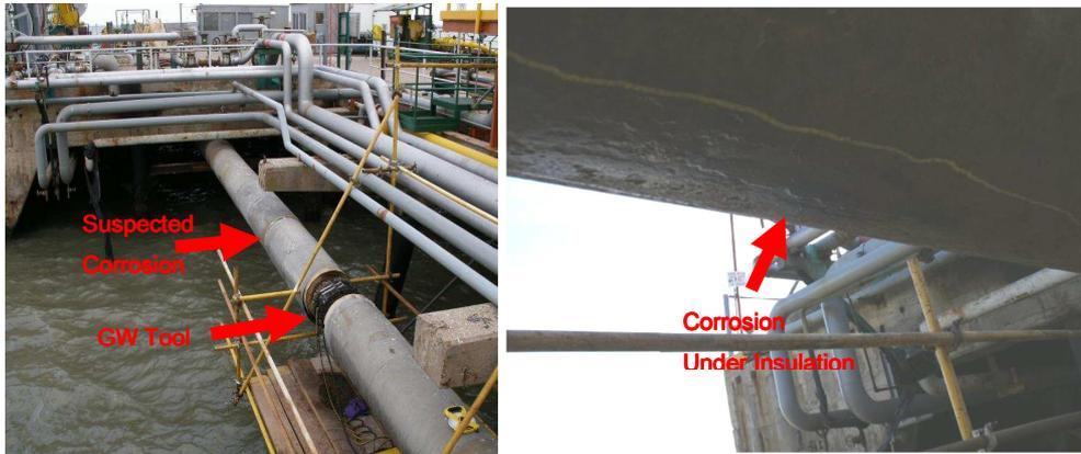
**Figure 1.1: Jetty Line Inspection: - This area of corrosion under insulation was approximately 1 metre in length and 35% wall loss and was detected by Guided Waves. The cost of inspection would be significantly higher to inspect the length of this pipe using localised NDT methods due to scaffolding provisions for access and the unnecessary removal of protective insulation.**
