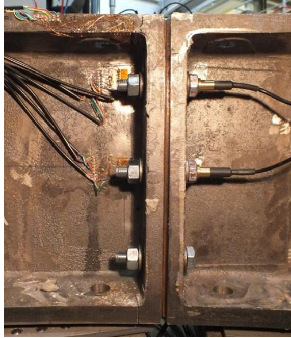
(a) Upper and lower circumferential flange fracture in segment J
