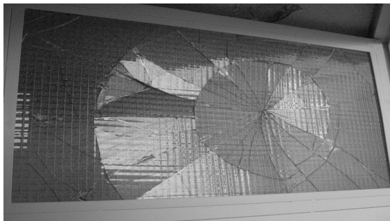
Fig. 6: Recently replaced window on the door of a rehousing building.
