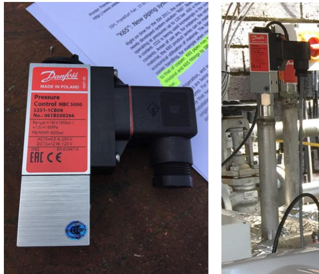
Figure 6.8 Photographs of pressure control switch
