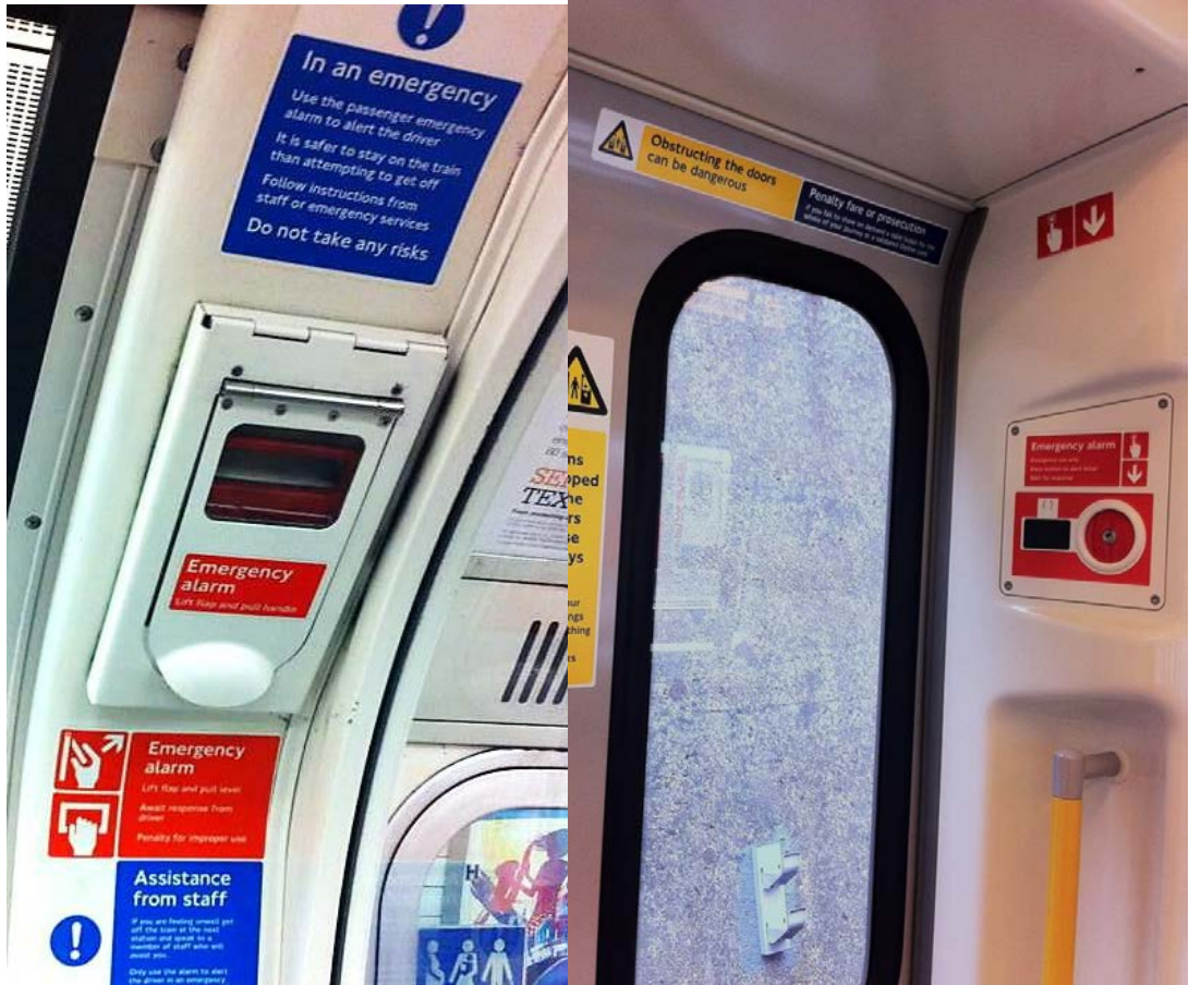
Figure 4.11 (Left) Emergency alarm at doorway in the Victoria line train
