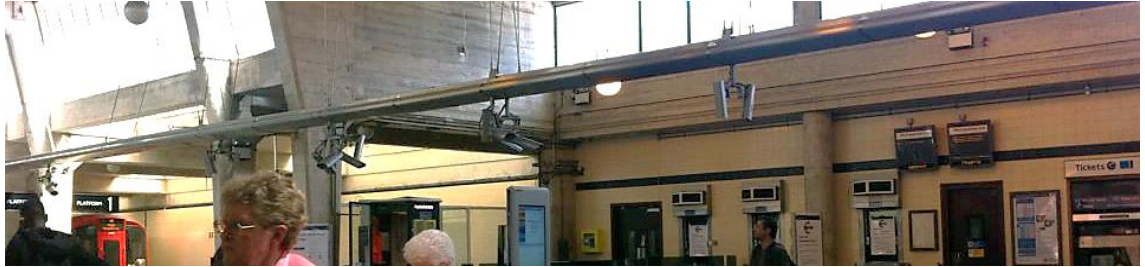
Figure 4.5 CCTV cameras installed at Uxbridge station ticket hall
