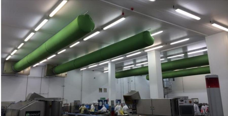
Figure 3-16. Case study 2: Air distribution system via circular fabric ducts
