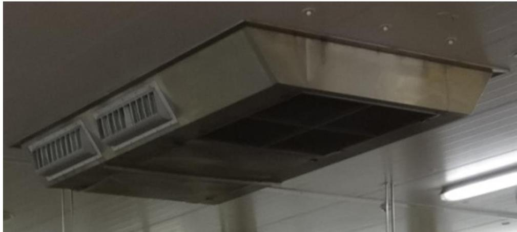
Figure 3-4. Case study 1: Air distribution system via supply/return diffusers.
