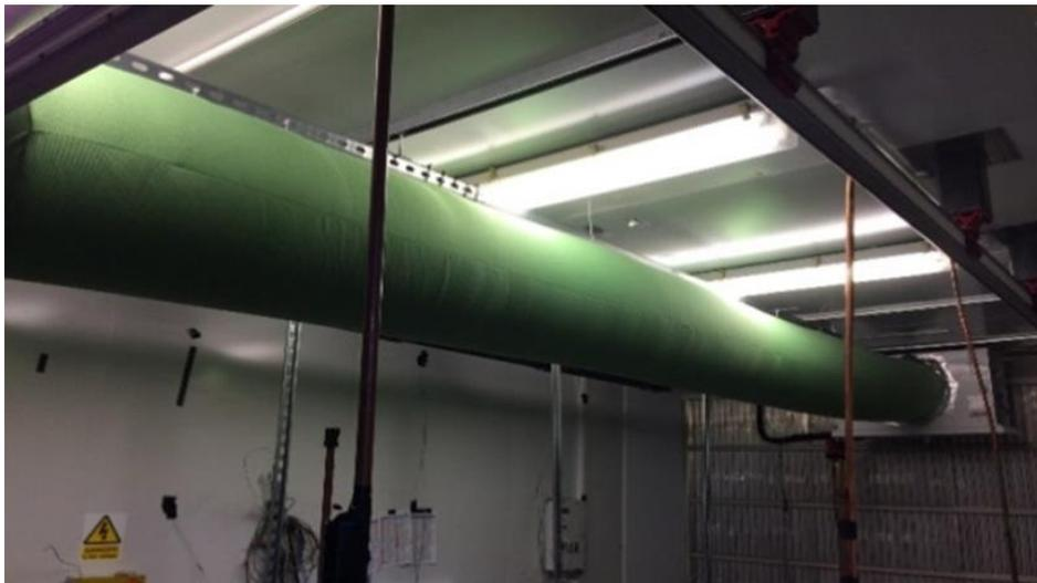
*Figure 4-3. Experimental test facility: Air distribution via circular fabric duct.*
