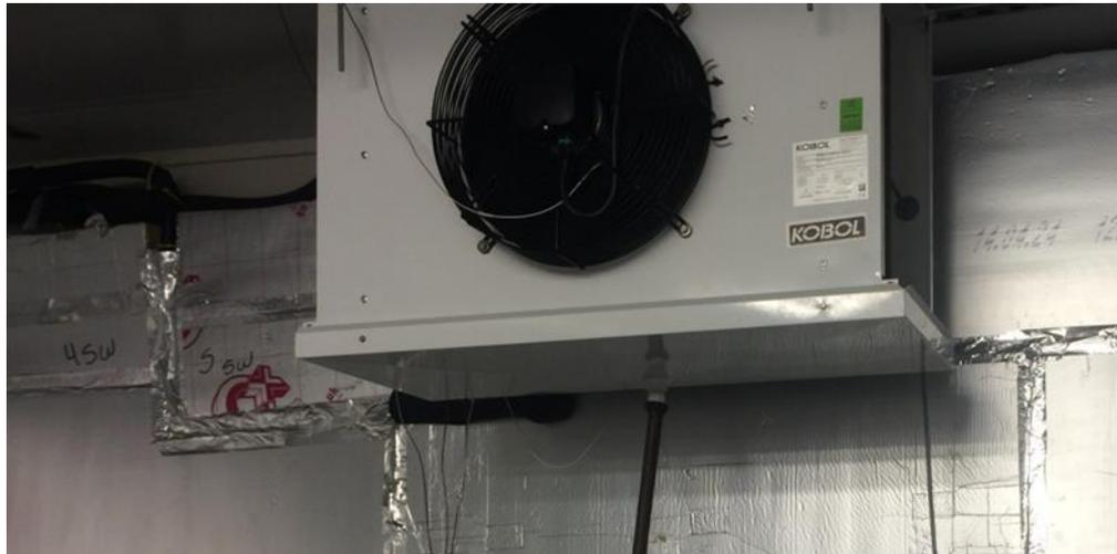
*Figure 4-15. Experimental test facility: Air distribution via non-ducted evaporator coil*
