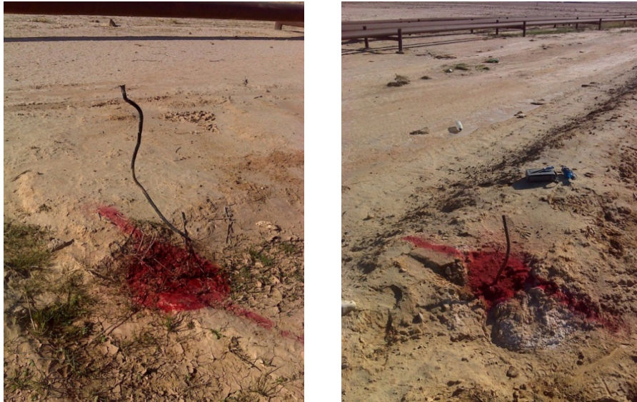
Figure 4-10: Part of the Metal Rod for the Sacrificial Anodes (no longer present) Attached to the Pipe via a Tack Weld
