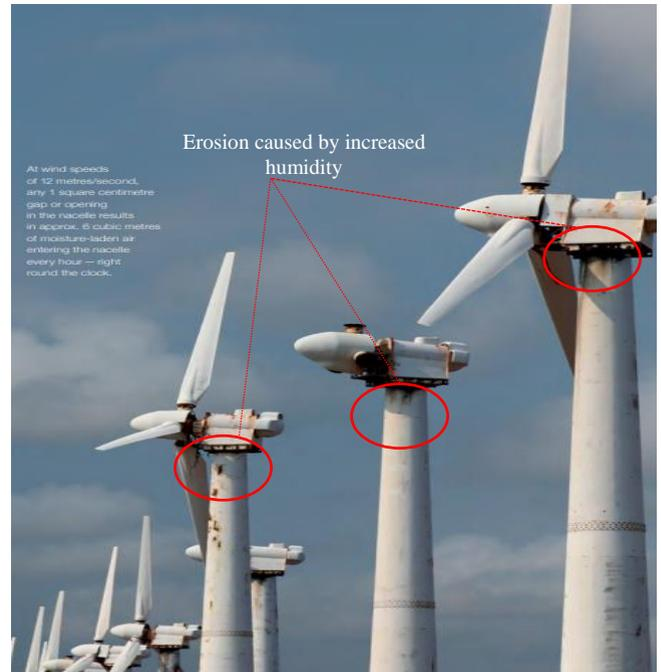
FIGURE 19. Humidity effect on wind turbines
