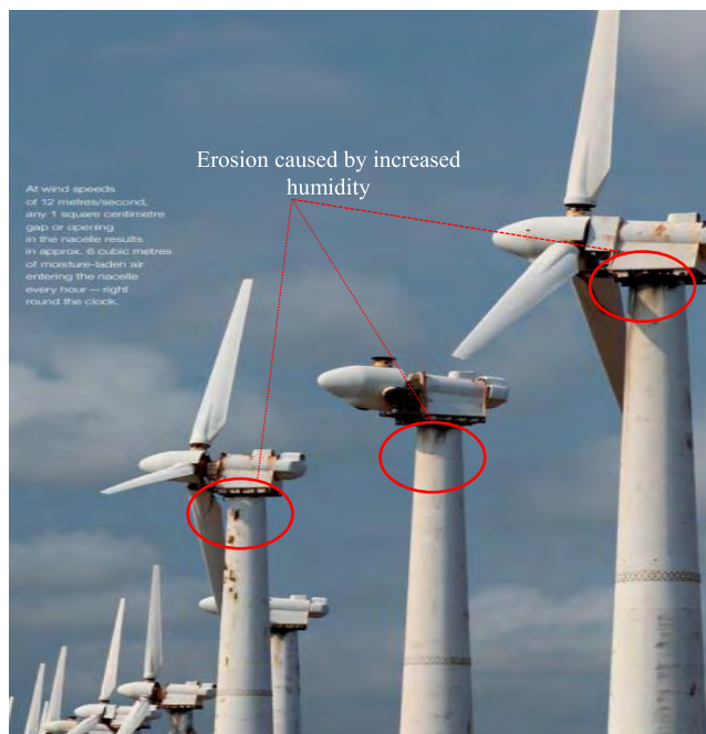
FIGURE 19. Humidity effect on wind turbines.
