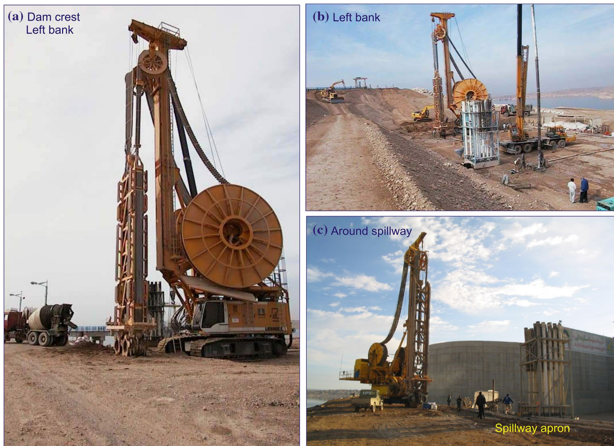
Fig. 4 The BC-40 trench-cutter working at various part of the Karkheh dam during the construction of the complementary cutoff wall
