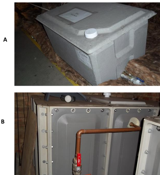
Figure 1.11 Single piece factory insulated moulded GRP cold water storage tank (A) and sectional factory insulated GRP cold water storage tank (B) . (Source: own collection)
