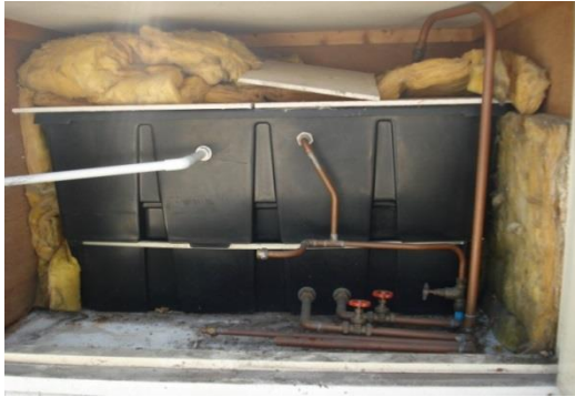
Figure 1.16a. Single piece plastic tank without clear space around (Source: own collection)
