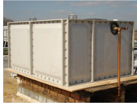
Figure 1.16b. Pre-insulated GRP sectional tank with clear space around
