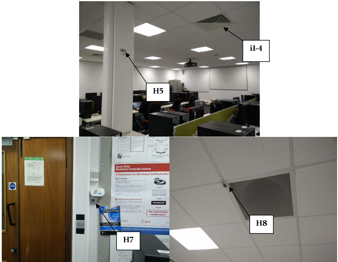
Figure II.1 – Seminar Room view with the location of two sensors, wall mounted control and H7 and HOBO (H8) placed at the exhausting griddle.
