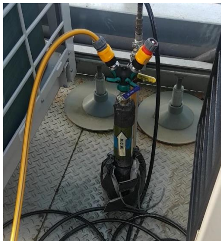
Figure 5.31. Pipe connection to tap water supply and 2-way manifold
