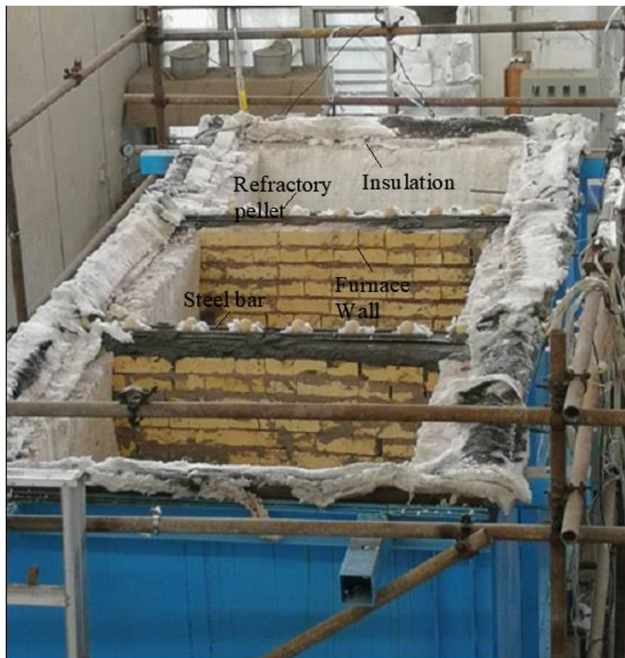
(b) Photograph of the internal wall
