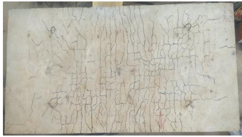
(a) Cracking pattern on the top surface
