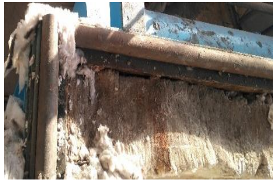
(b) Steel roller on the external furnace wall
