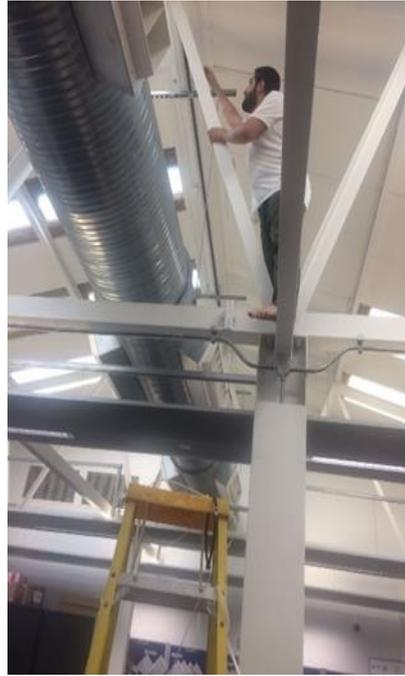
Figure 4.14 HOBO Temp/RH data logger mounted on the unoccupied zone
