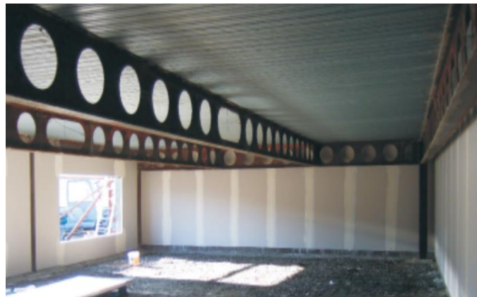
Fig. 0.2 Fire test conducted by the University of Ulster (Nadjai et al. 2011)
