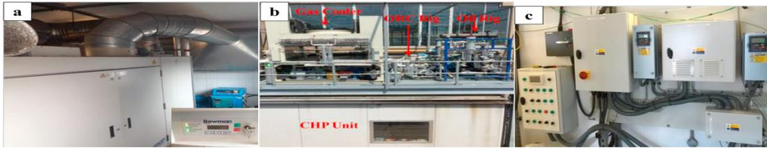
Fig. 2. Photographs of the system. (a) 80kWe CHP unit, (b) from view of whole system, (c)Recuperative ORC main control system.
