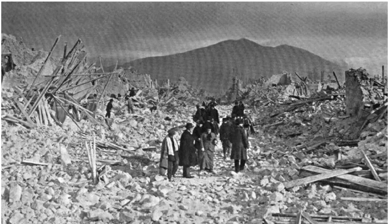
Figure 2. 1915 Avezzano earthquake – damage in Via Napoli [10]
