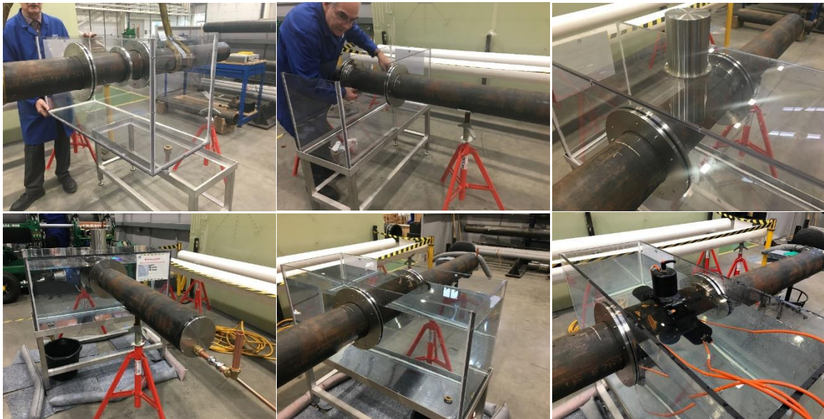
Figure 7.19: Assembly of the integrated system demonstration tank
