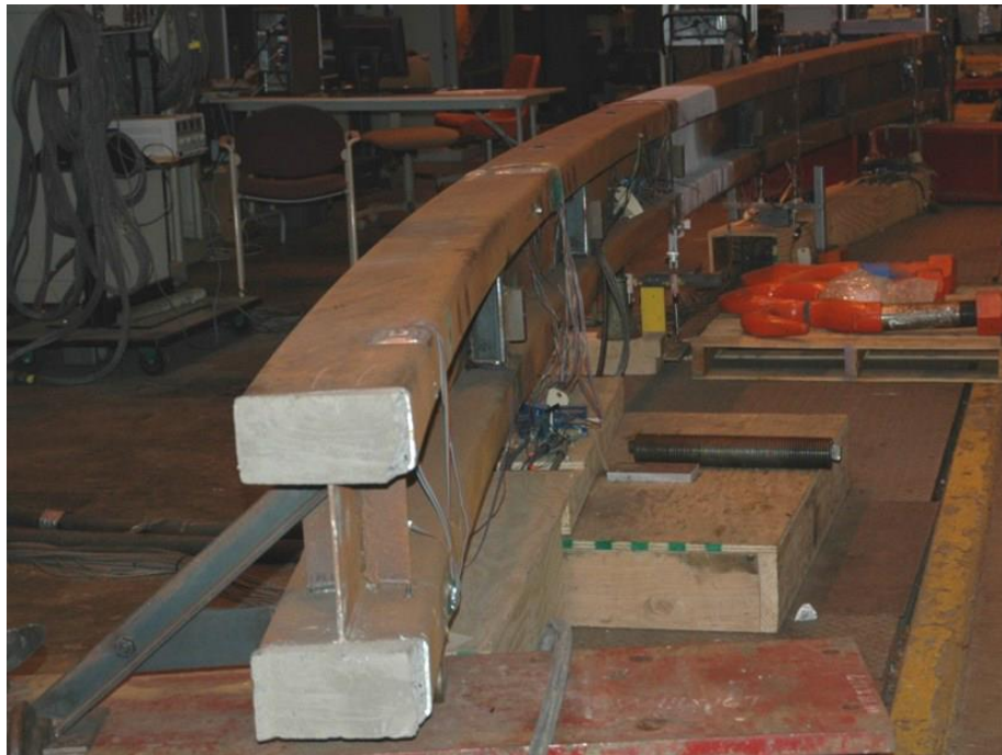
Fig. 2.23 Curved TFG with hollow steel tube flanges and concrete infilled ends (Putnam, 2010)
