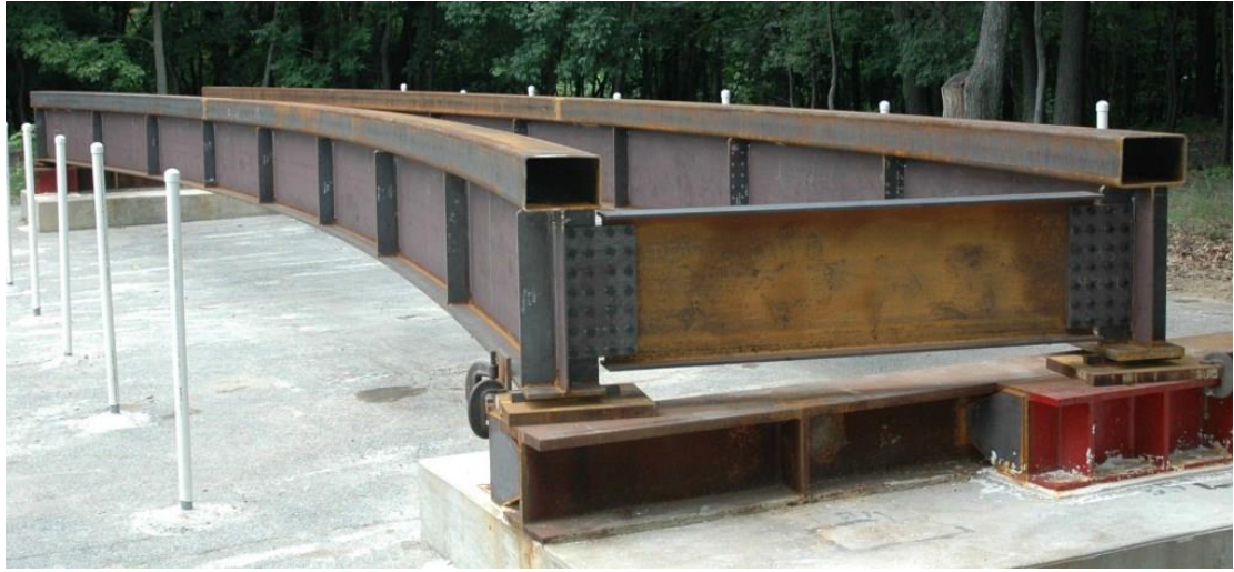
Fig. 2.25 Curved TFG with hollow steel tube top flange (Ma, 2014)
