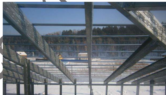
565 566 567 568 569 570 571 (a) Application of slotted perforated CFS channels
