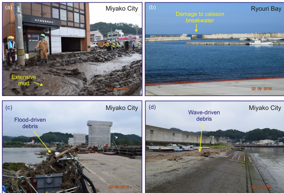
Fig. 3 Destructions made by typhoon Lionrock along the east coast of Japan in August–September 2016; Miyako City is indicated in Fig. 1, Ryouri Bay is located near Ofunato. Locations are: 141.9597° E and 39.6431°N for a; 141.8136° E and 39.0563°N for b; 141.9245° E and 39.6305°N for c; the location (d) is at a distance of a few hundred meters from location (c). Photographs belong to Mohammad Heidarzadeh
