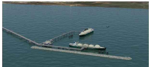
Figure 1 - Breakwater Protecting two berthed LNG vessels
