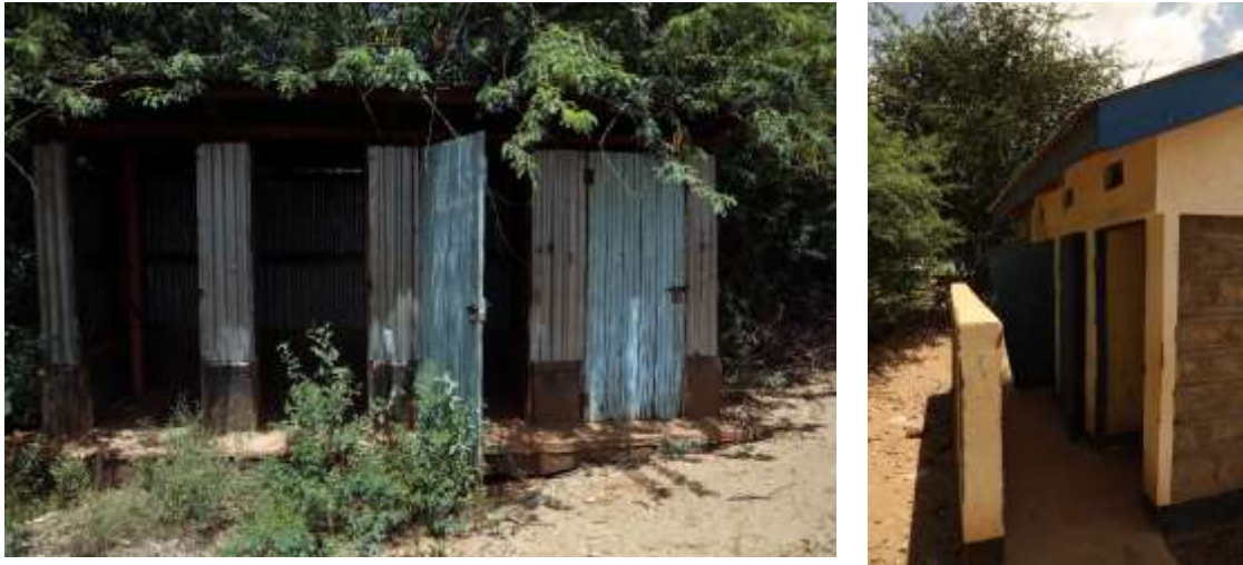
Figure 9-2: Old School Pit Latrines and new pit latrine block in Kakuma Refugee Camp in Kenya
