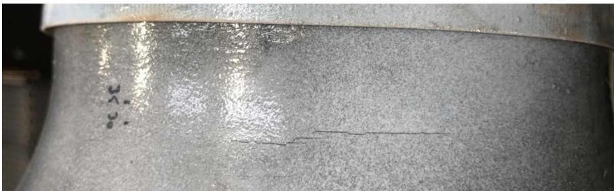
Figure 2-7 Visual inspection using a mobile camera
