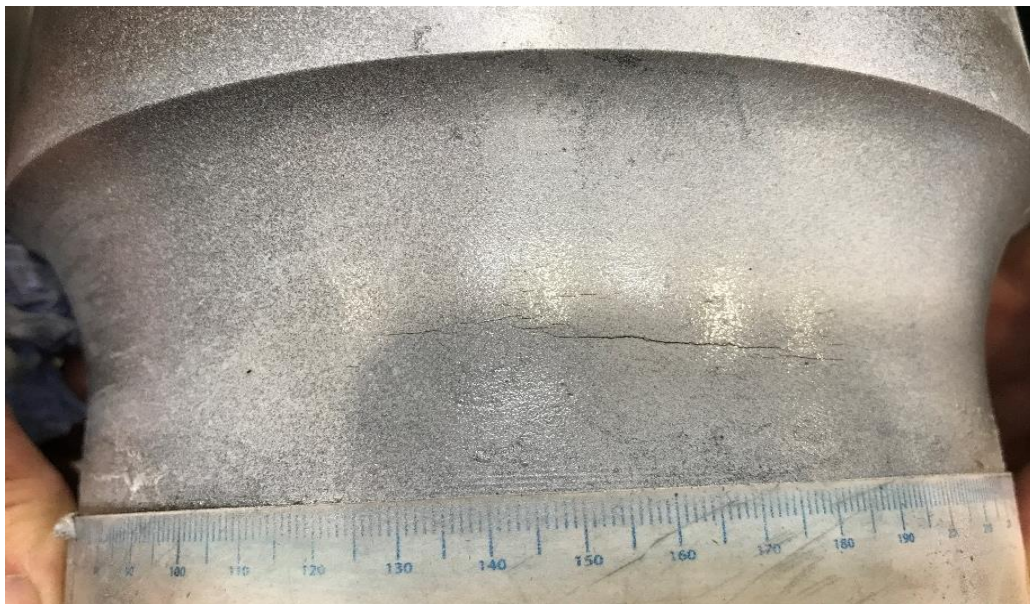
Figure 4-17 Image taken with a mobile of the 2 nd crack after using MPI
