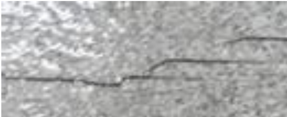
Figure 4-15 Magnified crack image at 9 th iteration showing improvement after applying MPI
