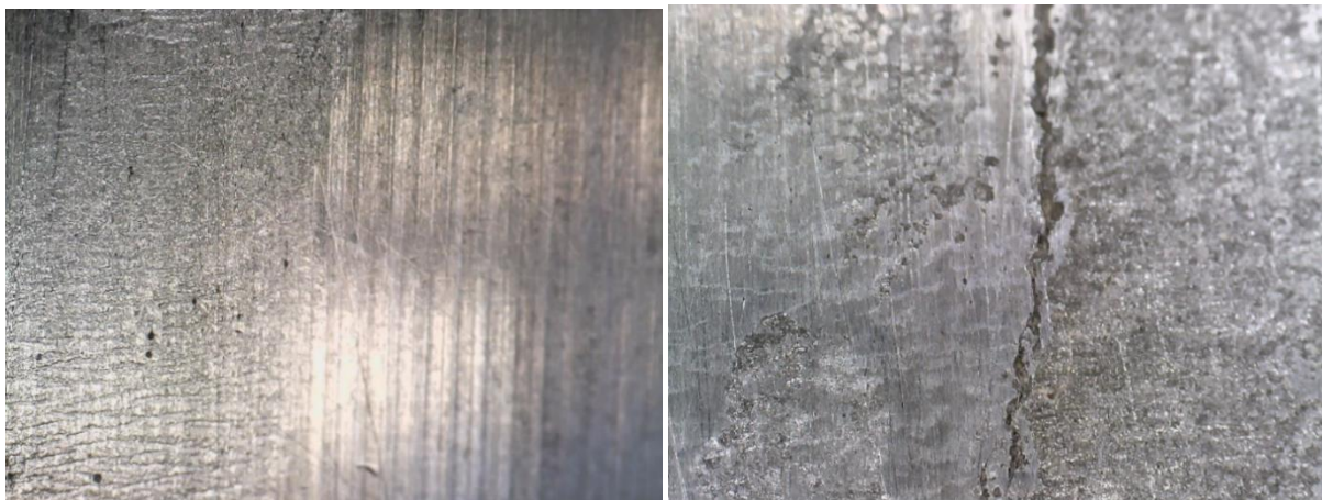
Figure 4-16 Image of 2 nd crack at 6 o'clock (a) at 2 rd iteration; (b) at 3 rd iteration
