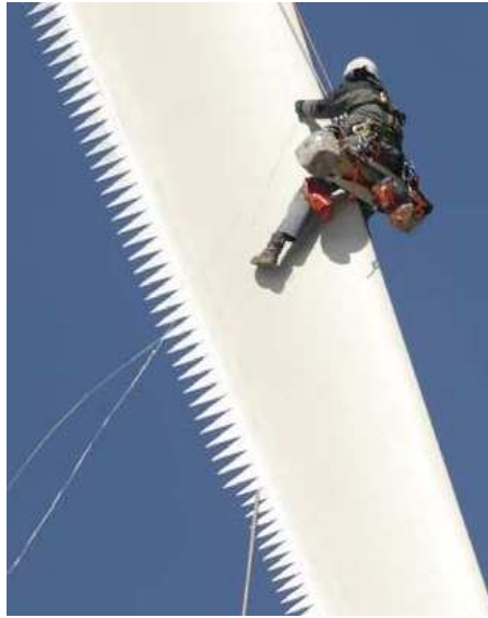
Figure 36: A typical MW-class wind turbine blade with serrations at the trailing-edge (Source: Oerlemans et al [223]).
