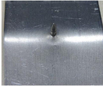
Figure 75 – Bottom view of interlock failure without any damaged to the element
