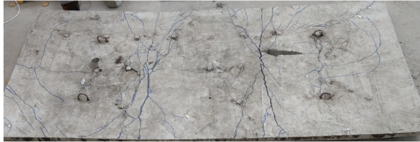
(a) Cracks on the top surface
