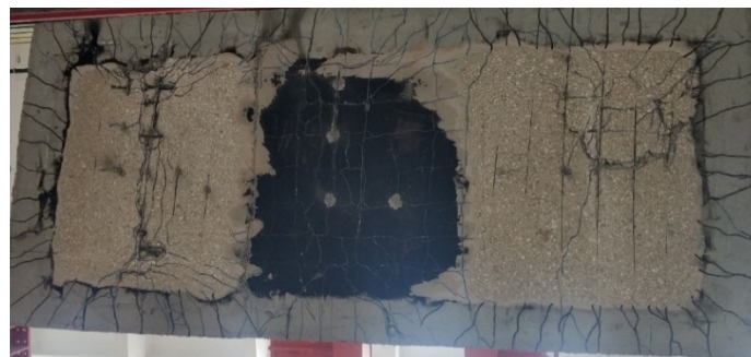
(c) Cracks on the bottom surface
