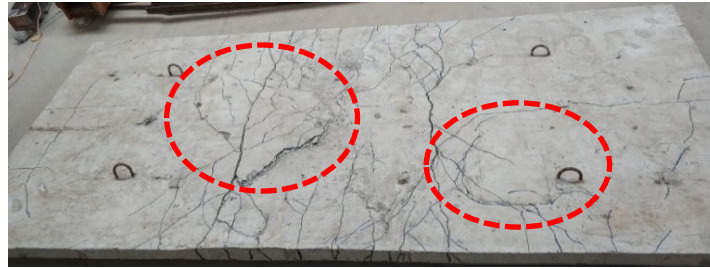
(a) Cracks on the top surface
