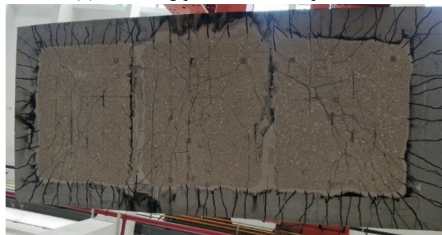
(c) Cracks on the bottom surface
