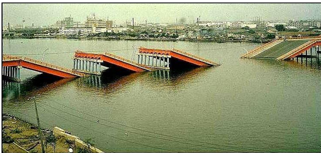
Figure 2-59 Collapse of Showa Bridge due to Liquefaction, (Yoshida et al. , 2007)
