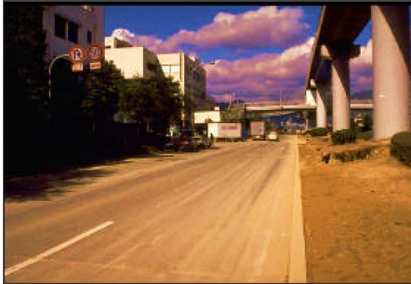
Figure 2-77 Differential Settlement of the Piers Supporting an Elevated Railway on Port Island, (Akia et al. , 1995)
