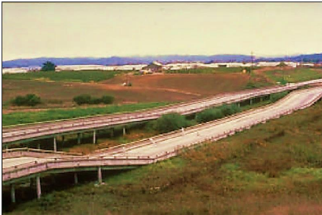
Figure 2-68 Collapse of Highway One Crossing Struve Slough due to Pile Punching Through Deck, (Seed et al., 1990)
