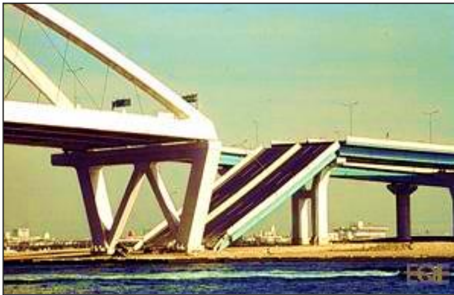
Figure 2-79 Collapse of the Nishinomiya Bridge Span, (Akia et al. , 1995)
