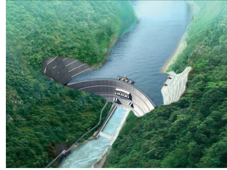
FIGURE 1: Survey of the Dagangshan Hydropower Station.
