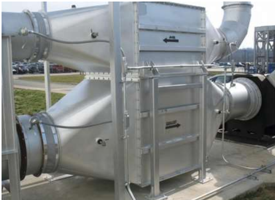
Figure 15: Photograph of a counterflow HPHE for an aluminium furnace [39].
