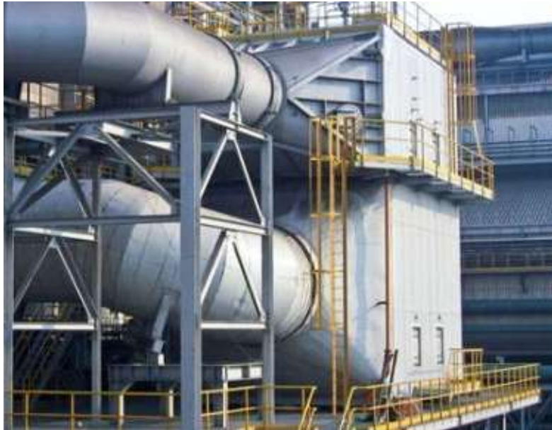
Figure 17: Photograph of an exhaust-to-coke gas HPHE unit [39].
