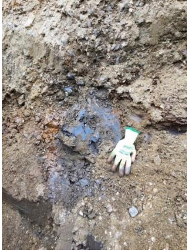
Figure 5. 32 – DFH infill at Battersea Power Station Phase 3. A large clay clast within the majority sand and gravel infill material. Exposure is approximately 2 m high and 1 m wide.
