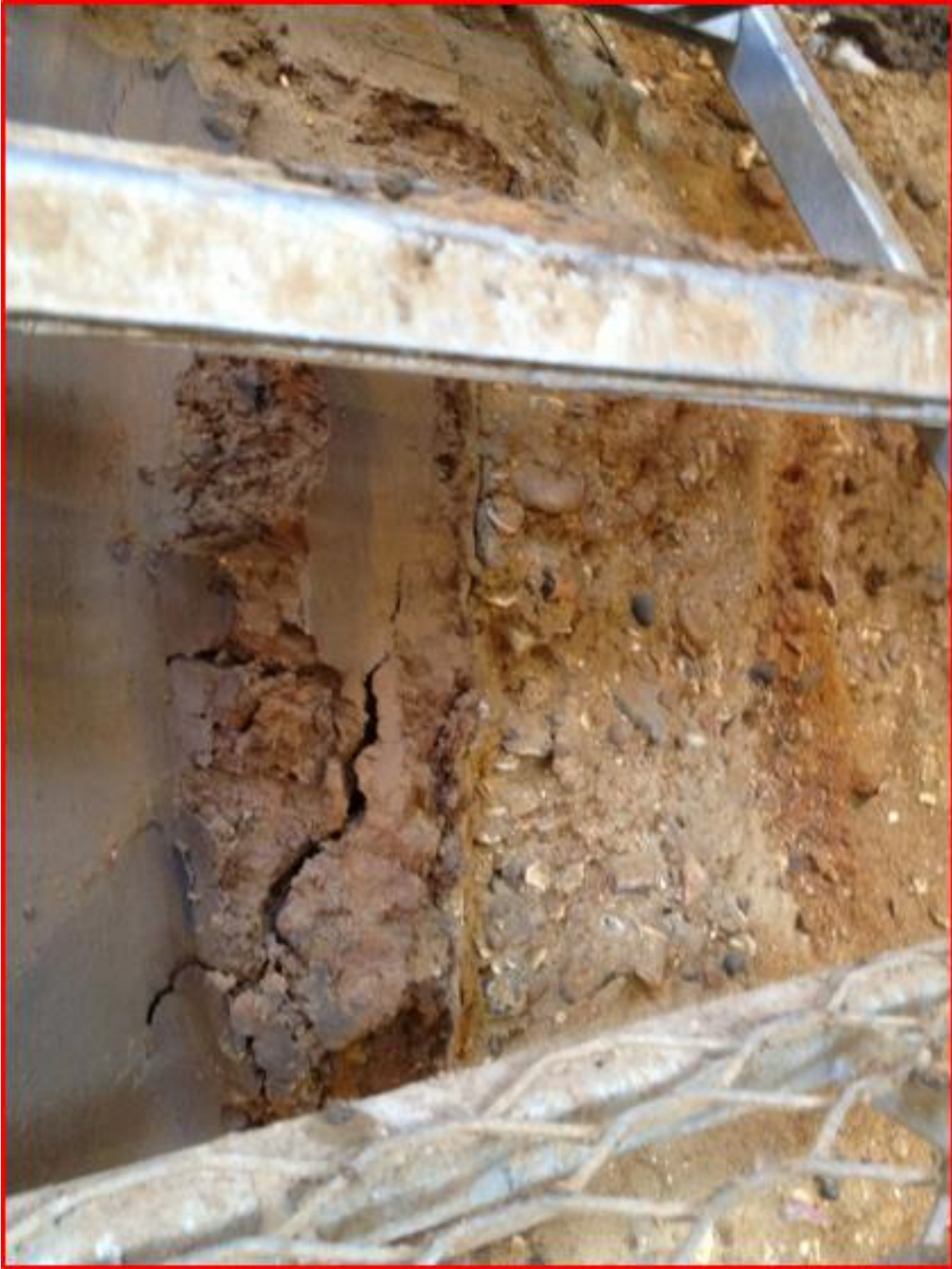
Figure 9.9 – DFH infill showing vertical contact between clay, mixed deposits and oxidized, orange material to the right of the image.
