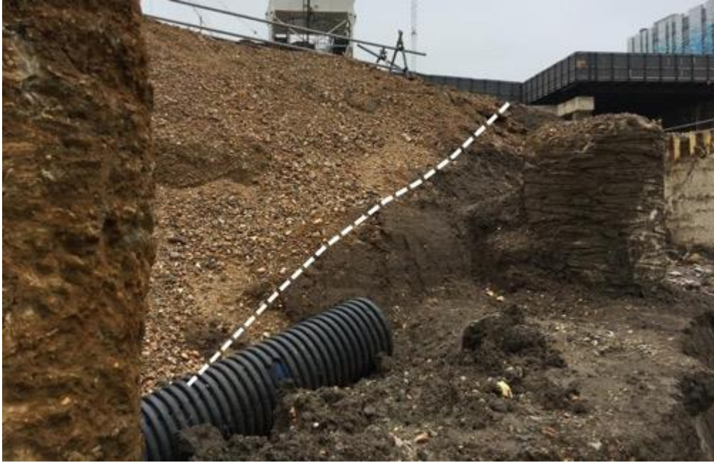
Figure 5. 27 – Photograph taken from within the excavation at Battersea Power Station Phase 3 showing the DFH infill contact with the London Clay. Note the gentle slope angle (around 40°) and the relatively sharp contact between the gravel infill and the clay beneath.
