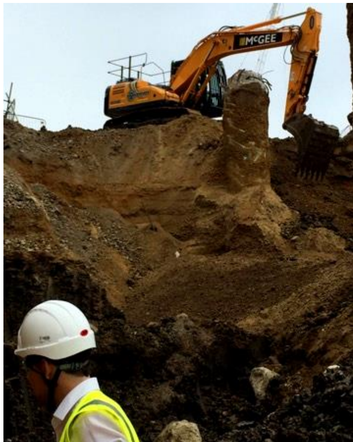
Figure 5. 28 – DFH infill at Battersea Power Station Phase 3. Undisturbed horizontal horizons are identifiable within the sand and gravel infill beneath the excavator.
