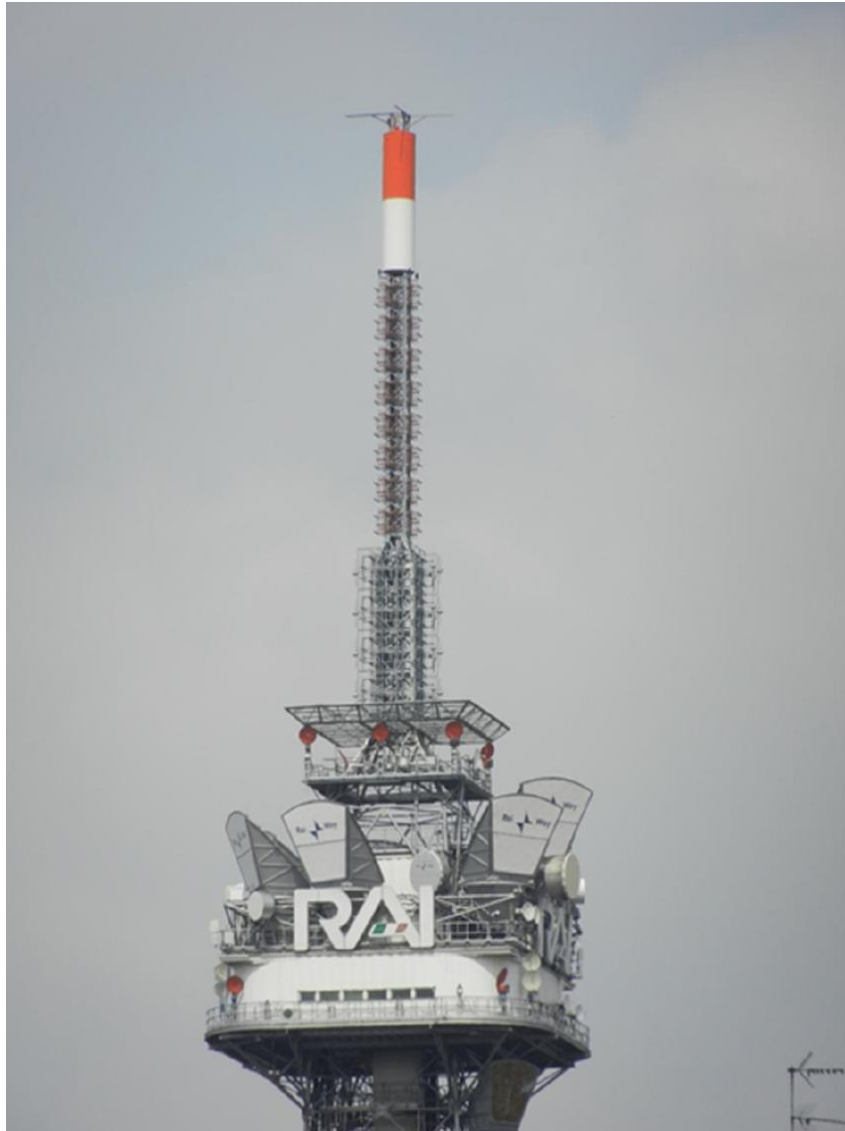
Figure 25. Antenna tower with a collinear array in the city of Milan, Italy
