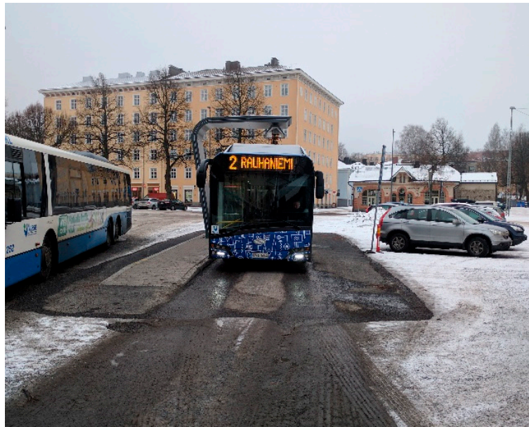
Figure 12. Heated foundation for the charging point to remove snow build-up on driving tracks.
