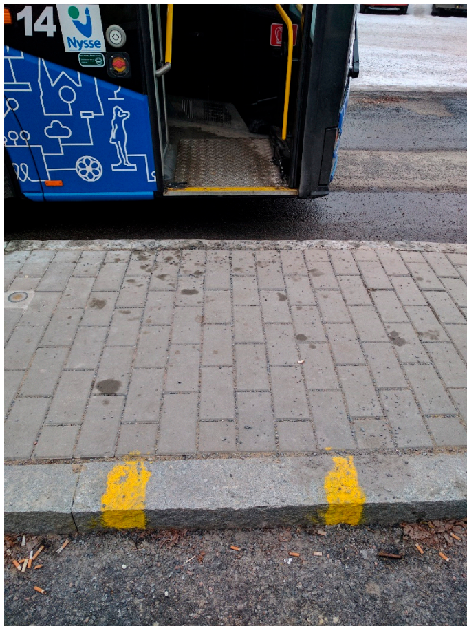
Figure 13. Paint markers on the kerb to position the bus for charging.
