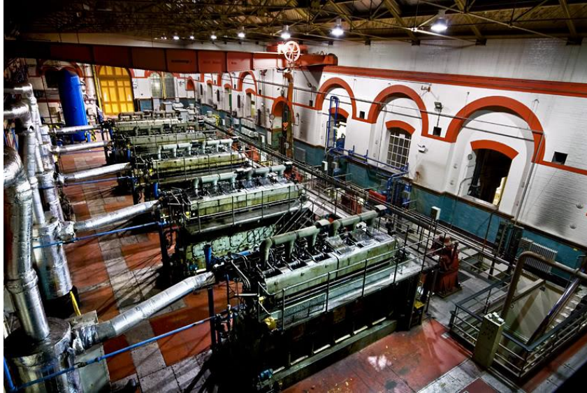
Figure 2-13 Lots Road Storm Sewage Pumping Station [76]
